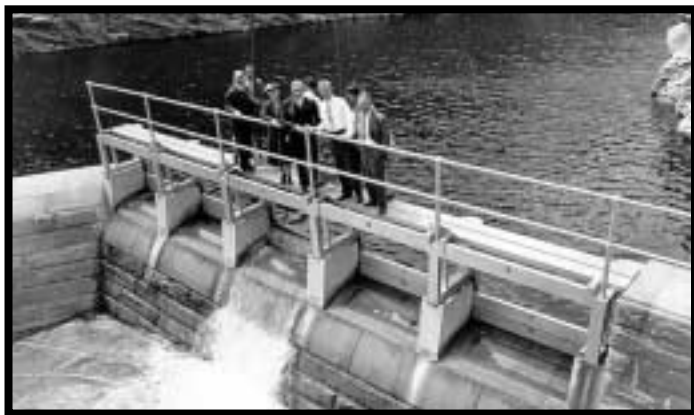
June 22, 1946: Engineers and officials along with Mrs. Frank Winsor, widow of the Chief Project Engineer, were on hand when stoplogs were removed from the Spillway Wall releasing the first Quabbin water down the Spillway Channel.
